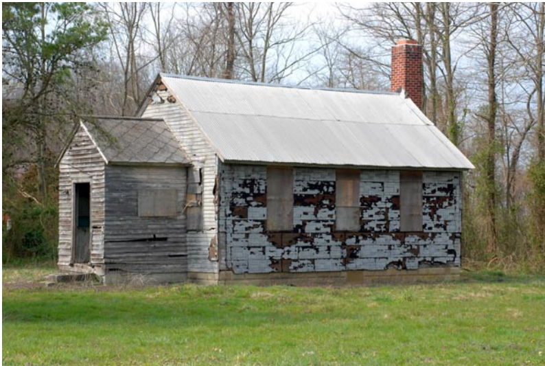
Marshalltown Historic District, Mannington Township, Salem County
