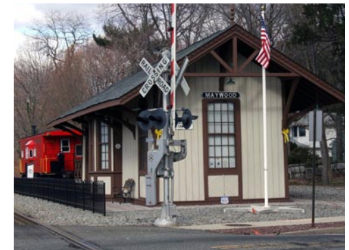
Maywood Railroad Station, Maywood Borough, Bergen County
