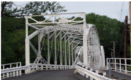
Elm Street Bridge, Hillsborough & Branchburg Townships, Somerset County
