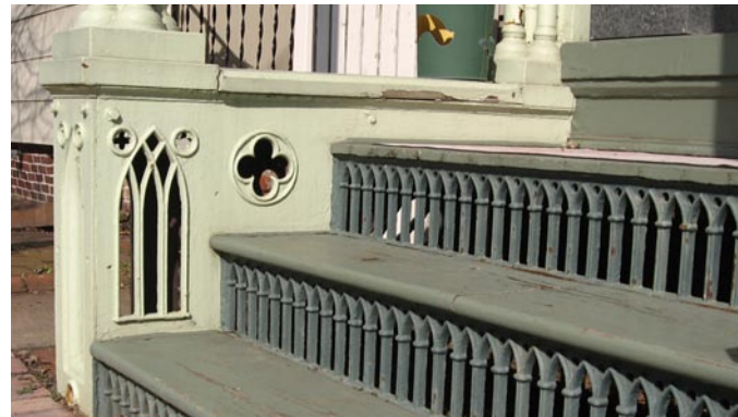
Gothic Revival Stoop, Bordentown City, Burlington County
