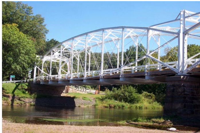
Lenticular Truss Bridge, Neshanic Station, Hillsborough & Branchburg Townships, Somerset County
